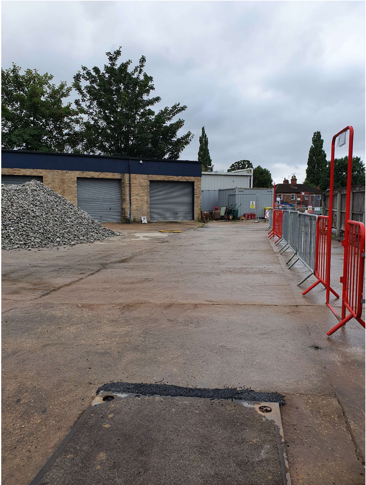
Within the site
